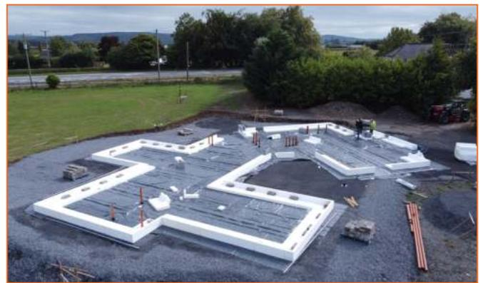
After an initial ground investigation survey on-site, the footprint of the building + 1m is excavated down to good natural ground. Graded stone fill (typically T3 blinding on T2 permeable on T3 structural) is placed and compacted with services installed as per the project engineer's instructions. The radon membrane is fitted on top of the T3 blinding prior to assembly of the insulated raft, at a later stage the membrane is dressed up the outside of the insulated raft.
