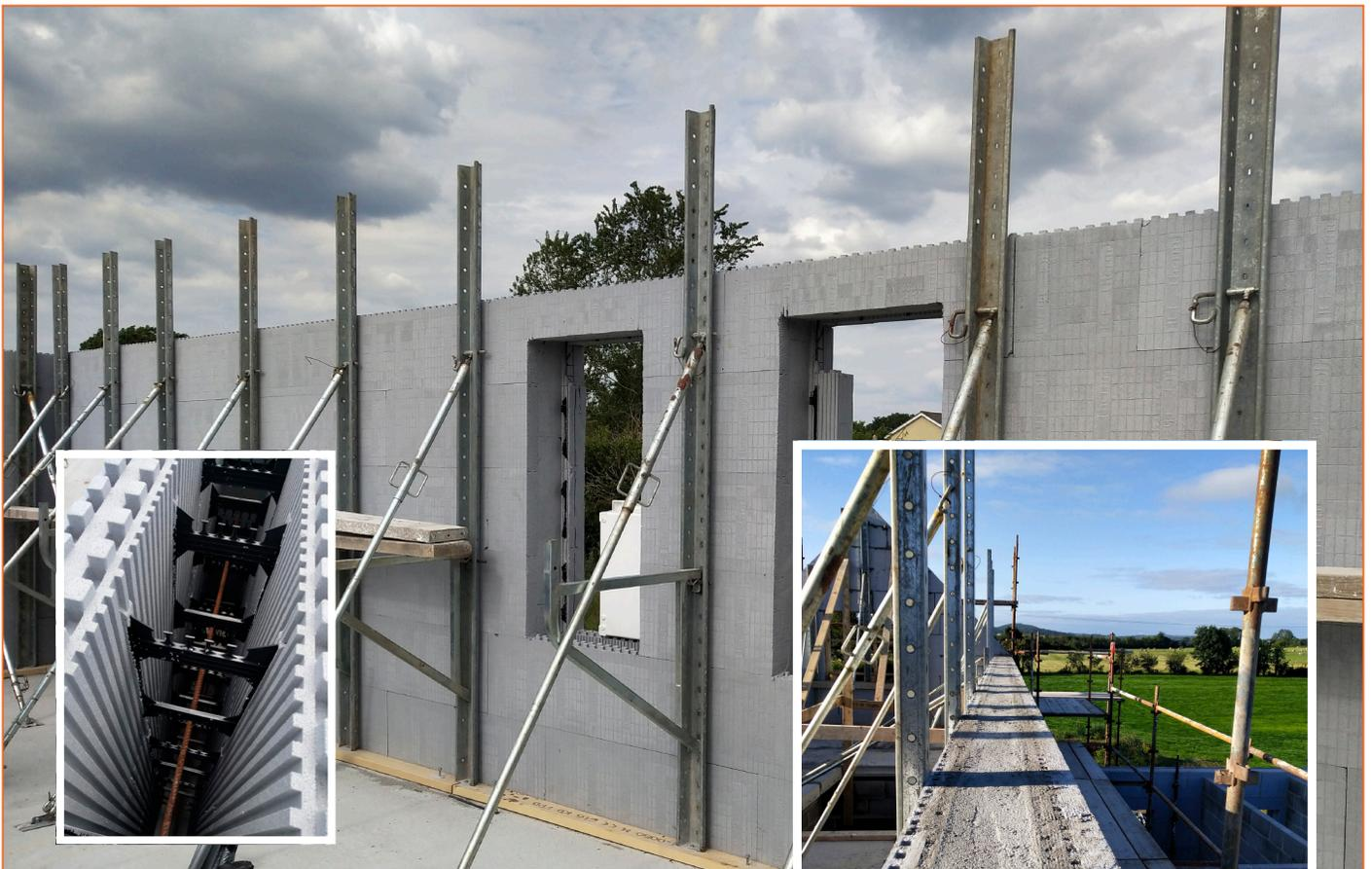
ICF-Therm polystyrene blocks are assembled on-site to create a formwork wall into which horizontal and vertical steel reinforcement are fixed for extra strength. Once braced, the formwork is then filled with readymix concrete. The ICF-Therm blocks remain in place permanently to create a super-insulated monolithic concrete structure.
