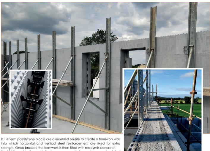
The ICF-Therm blocks remain in place permanently to create a super-insulated monolithic concrete structure.
