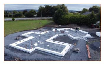
After an initial ground investigation survey on-site, the footprint of the building + 1m is excavated down to good natural ground. Graded stone fill (typically T3 blinding on T2 permeable on T3 structural) is placed and compacted with services installed as per the project engineer's instructions. The radon membrane is fitted on top of the T3 blinding prior to assembly of the insulated raft, at a later stage the membrane is dressed up the outside of the insulated raft.
