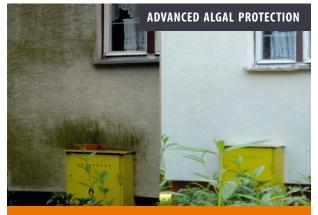
One coat of the silicone render contains biocides which provide a robust antimicrobial coating to your walls.
