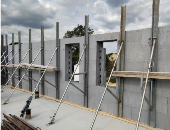
Figure 3: Bracing System for Castleforms ICF Therm Walls
