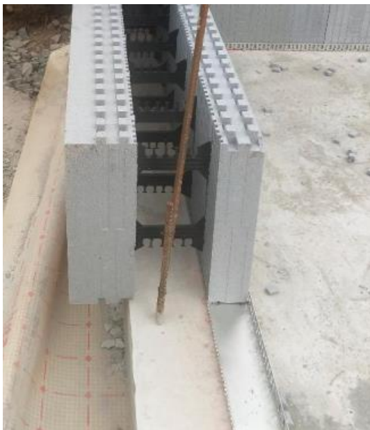
Figure 2: Castleforms ICF Therm Wall and Starter Track
