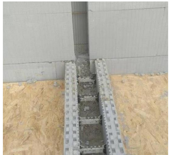
Figure 1: Construction of Compartment Wall
