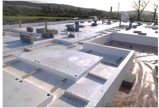
Figure 1 - Castleforms Raft Therm EPS Components
